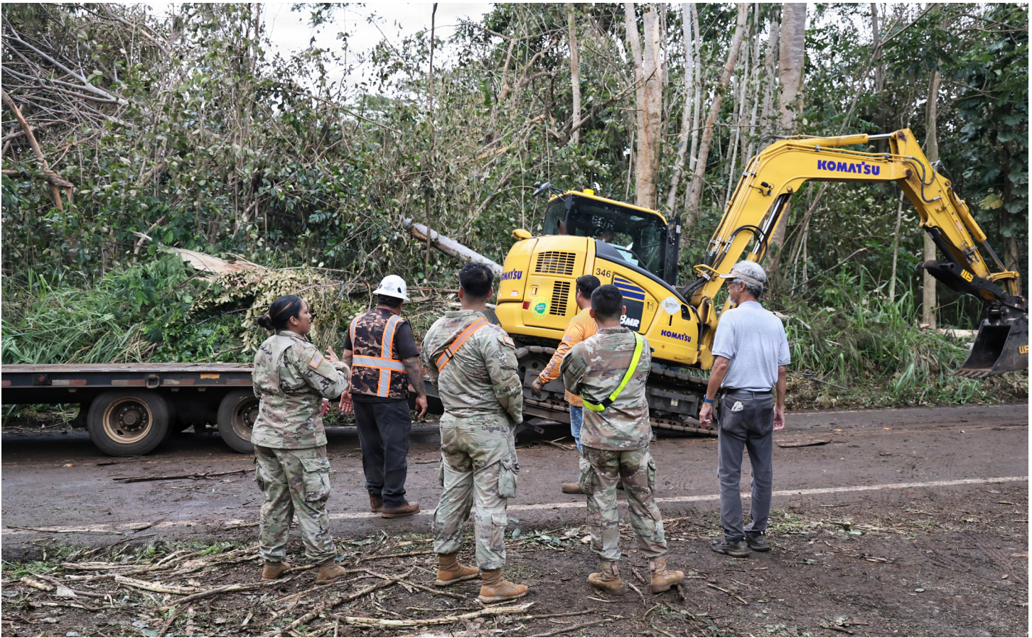
Members of the Hawai'i National Guard's Task Force Kaua'i assisted with debris cleaning in Kapa'a on Sept. 10. The Hawai'i National Guard was actively supporting state and county recovery efforts on Kaua'i from Hurricane Lowell, while simultaneously continuing recovery operations from Tropical Storm Lala on the Big Island. (U.S. Army National Guard photo by Staff Sgt. Randall Corpuz)
