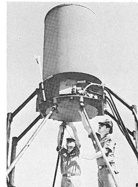
CMSGT Walter Furuyama and SSGT Roy S. Yamasaki complete the TACAN adjustments.
