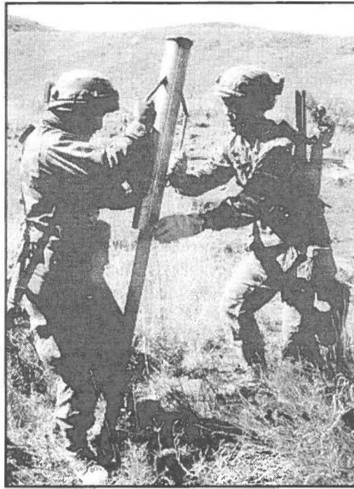
2nd Lt. Jeffrey D. Hickman SECURITY POSTING — Pfc. Gregory D.L. Auna and Sgt. Ryan H. Goto, from the 227th Engineer Company, pound post for barbed wire perimeter fighting positions.
