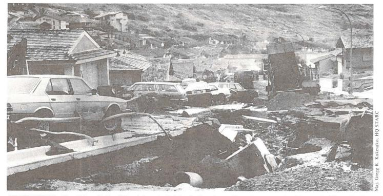
TEAM EFFORT—Hawaii Army National Guard dump trucks bring in dirt and gravel for a city contracted bulldozer to level into a deeply eroded Kahena Street that was washed out by flood waters. The temporary road enabled cars and debris to be cleared off the Nui Valley street which had become a wasteland during the New Year's flood.
