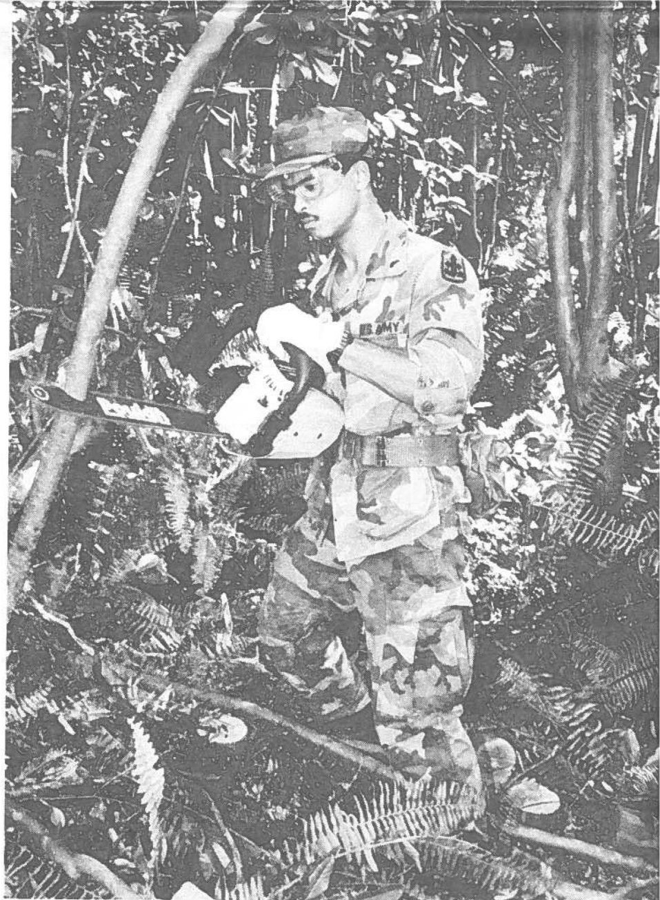
TRAIL BLAZER —Hawaii Army National Guardman Sgt. Clayton Calarruda uses a chainsaw to clear over growth on Okolehao Trail in Hanalei, Kauai. The 227th Engineer Company worked with the State's Department of Land and Natural Resources to select sites that were within the trscope of the Army engineers.
