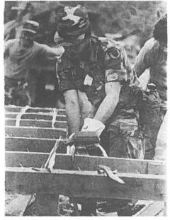
I SAW WHAT I SAW—Private Paul Amigable, 227th Engineer Company, HARNG, uses the chain saw to prepare the framework for the footbridge under construction. (Photo by 1st Lt. Curtis Matsushige, 117th PAD, HARNG)
