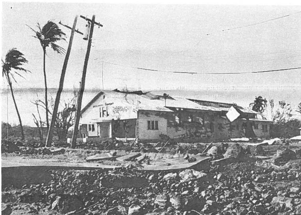
ARMORIES HIT —The Hanapepe Armory was among the several Guard buildings damaged by Hurricane Iwa. The Kapaa Armory was supposed to be an evacuation center, but heavy damage forced evacuees to other sites.
