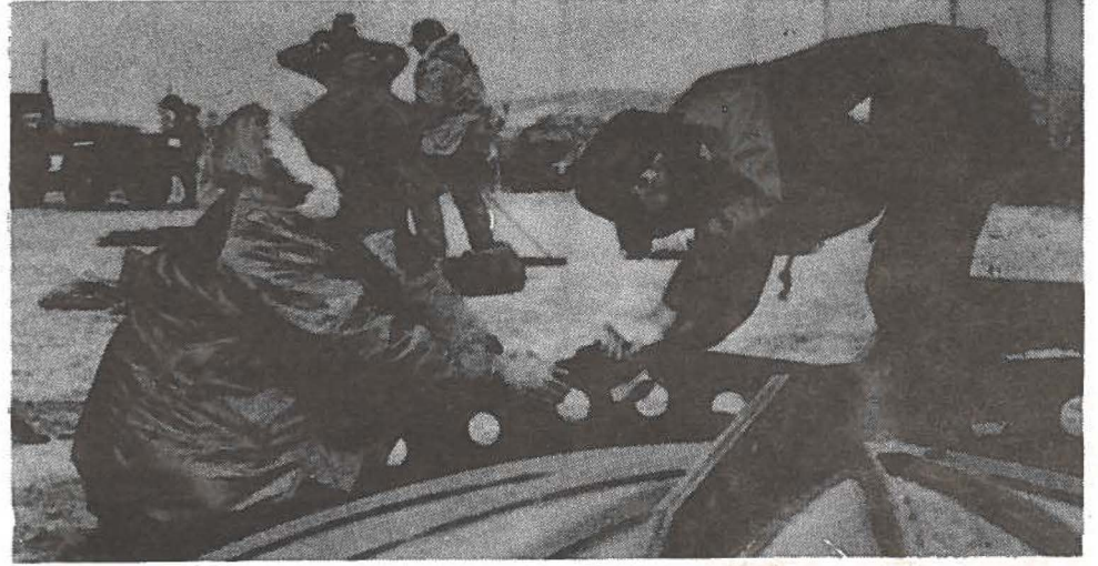
BRAVING THE COLD OF KOREA — SSgts. Edward Omine and Wallace Kakemoto assemble the 201st's TRC-97 antenna reflector during their recent trip to Korea. — Photo by Maj. Ernest Shima
