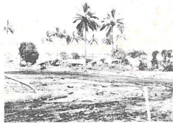
Damages to Hilo after tsunami of May 23, 1960.
