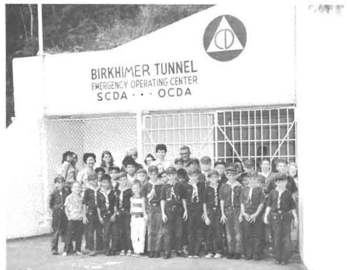
TOUR TUNNEL — This Cub Scout group from Pack 247 in Kailua was one of the many organizations that toured the Civil Defense emergency operating center in Birkhimer Tunnel during the year.
