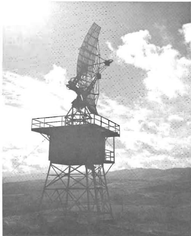
ELECTRONIC SENTINEL —A height-finding radar of the Hawaii Air National Guard scans the skies over the Hawaiian Islands. It is one of many Guard radar installations helping to protect our state.
