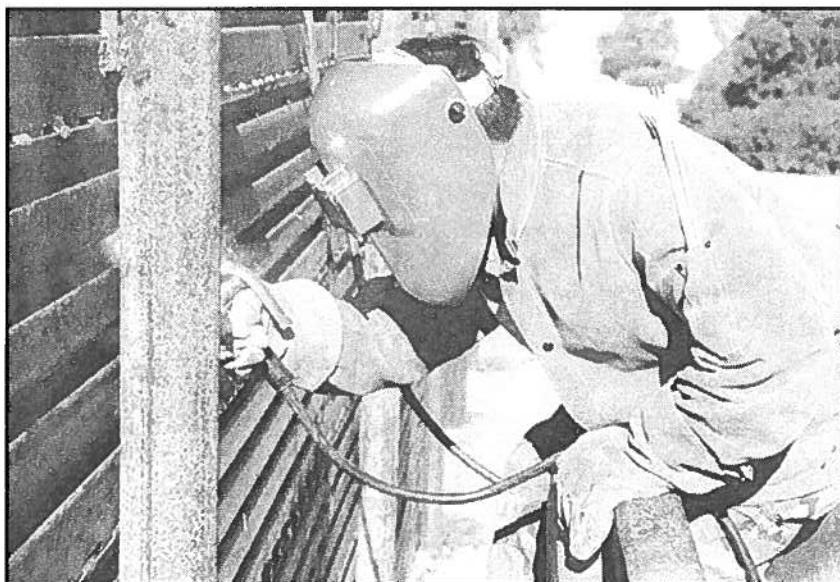
WALL LOCKER — An 227th Engineering Company soldier welds prefabricated landing mat into a 10-wall on the California-Mexican boarder. Spc. Brandon T. Bocanegra photo
