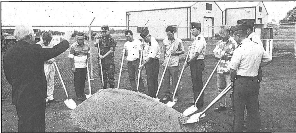
AVIATION FACILITY FOR THE NEW MILLENIUM — Rev. Charles L. Kahawai Sr. blesses the grounds of the new phase of the Hawaii Army National Guard Army Aviation Support Facility #2, January 1999. The expanded Hilo facility built on General Lyman Field will include a hanger, training offices and storage areas. Capt. Charles J. Anthony photo
