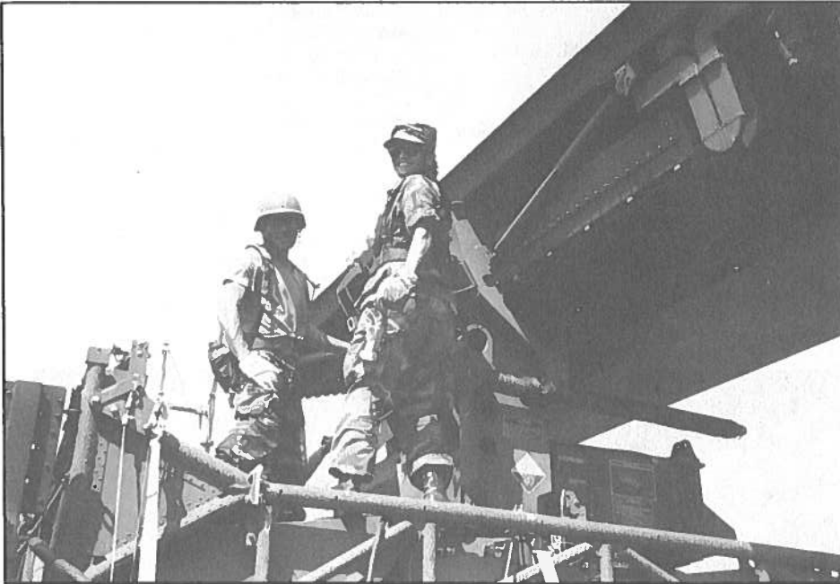
MOBILE COMMUNICATION -- Airmen from Kauai's 154th Air Control Squadron erect an antenna for the TPS-75 radar during a field training exercise at Mahaulepu, Kauai in early Spring 1994.
