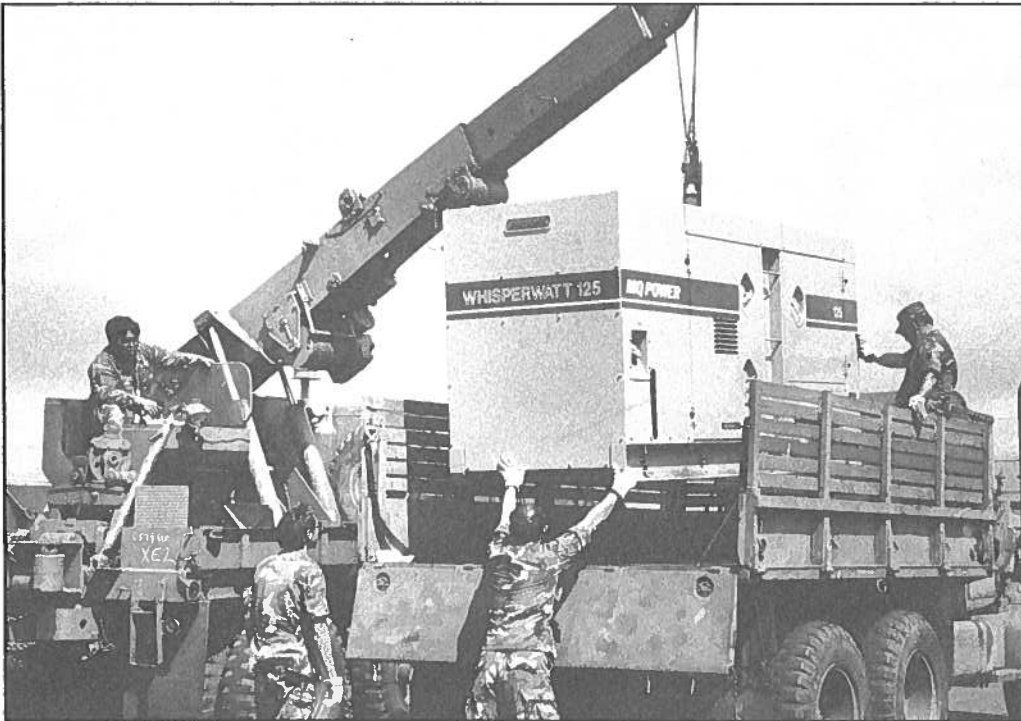
Airmen from Kekaha, Kauai's 154th Air Control Squadron load an emergency generator for delivery, May 18, 1993. The generators, on loan from the Federal Emergency Management Agency, were installed in schools, shelters and other priority sites.
