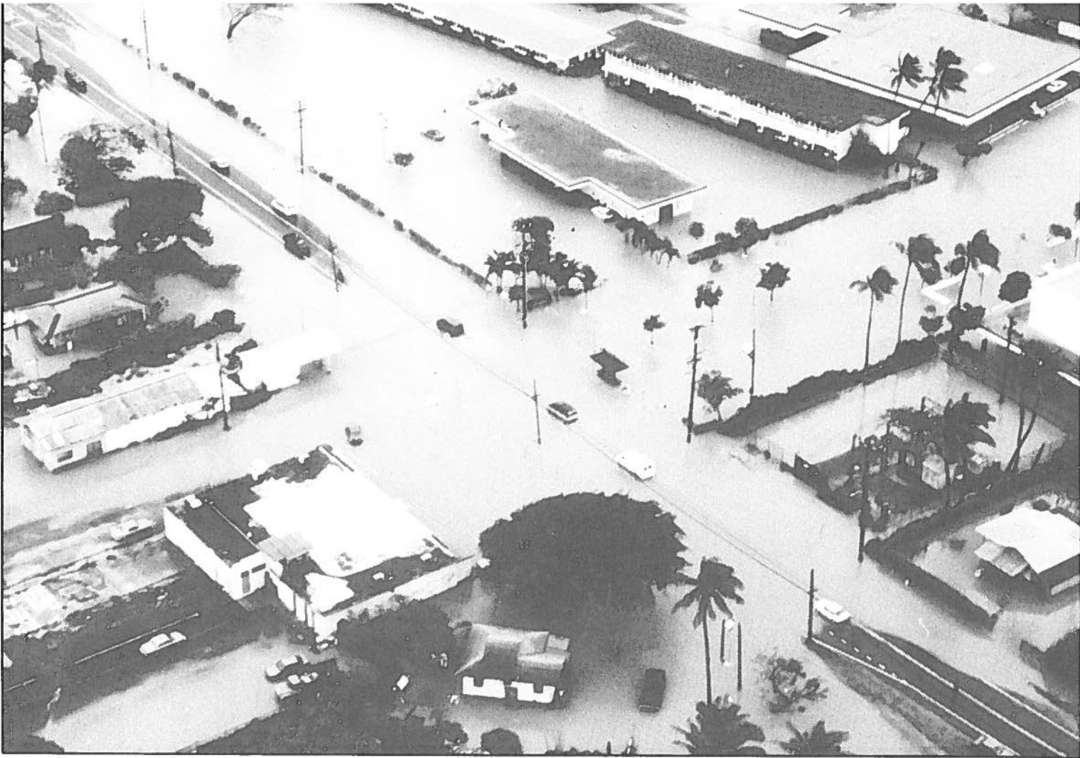
Kamehameha Highway in Kahuku, Oahu, was submerged by heavy rains, Mar. 19-23.
