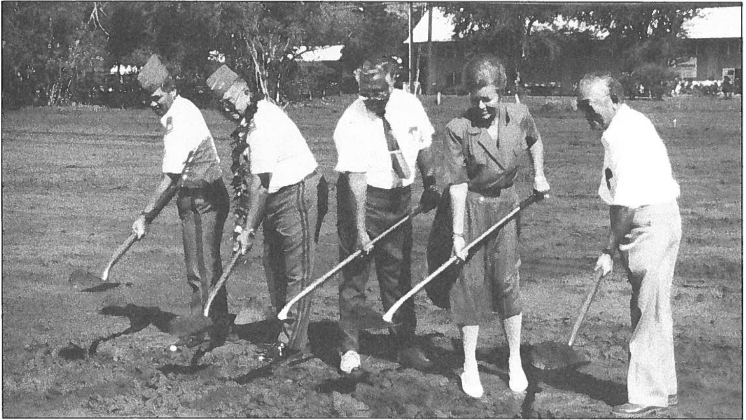
Ground is broken for Kauai's Hanapepe Armory, Oct. 11, 1988.
