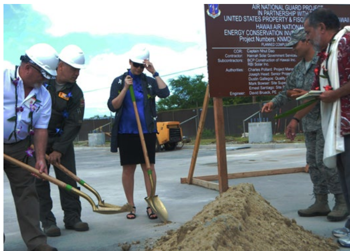
Retired U.S. Air Force Brig. Gen Stanley Osserman and U.S. Air Force Brig. Gen. Braden Sakai, Commander, 154th Wing, Hawaii Air National Guard prepare to shovel dirt at the ground breaking ceremony for a solar array farm being built for the HIANG at Joint Base Pearl Harbor-Hickam, Oct. 27, 2015. The solar array facility will be one piece of the HIANG's renewable energy strategy to decrease it's electricity expense and increase it's energy security. (U.S. Air National Guard photo by Senior Airman Orlando Corpuz/Released)
