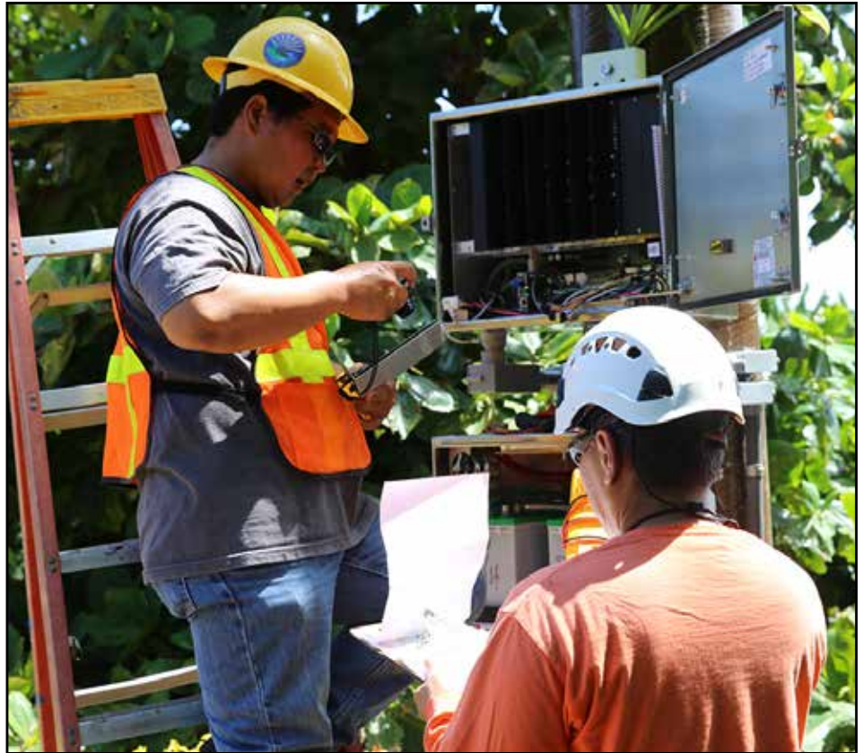
SOUND CHECK – Kurt Nagano and Jack Machida, SCD/HI-EMA radio technicians, inspect a siren installation at Camp Erdman, Oahu. Brian Miyamoto photo
