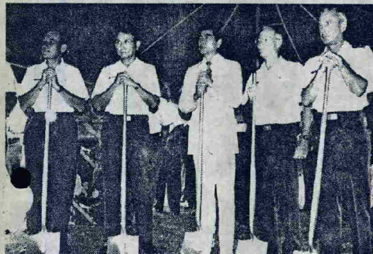
Governor Ariyoshi, center, appeared with PACAF and HANG leaders for HIROCC groundbreaking, Sept. 10.
