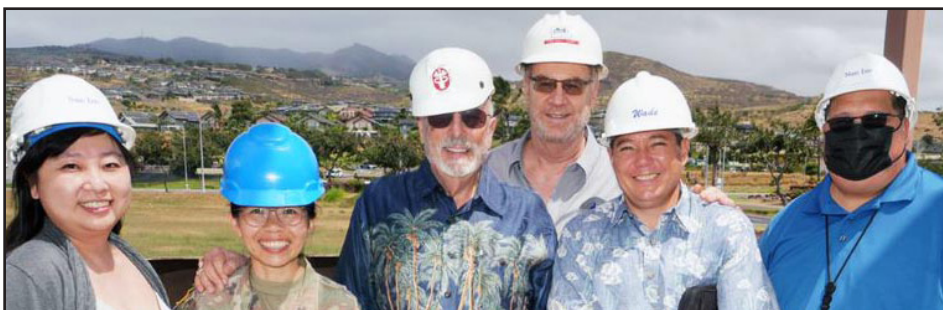
Yam Yi Lee, left, DOD Chief Engineering Officer Shaoyu Lee, Thomas M. Driskill Jr., DAGS Public Works Engineer/Project Manager Brad Leveen, DOD Engineer Wade Ishii and Ronald P. Han visiting the Daniel K. Akaka State Veterans Home in Kapolei on May 4, 2022.
