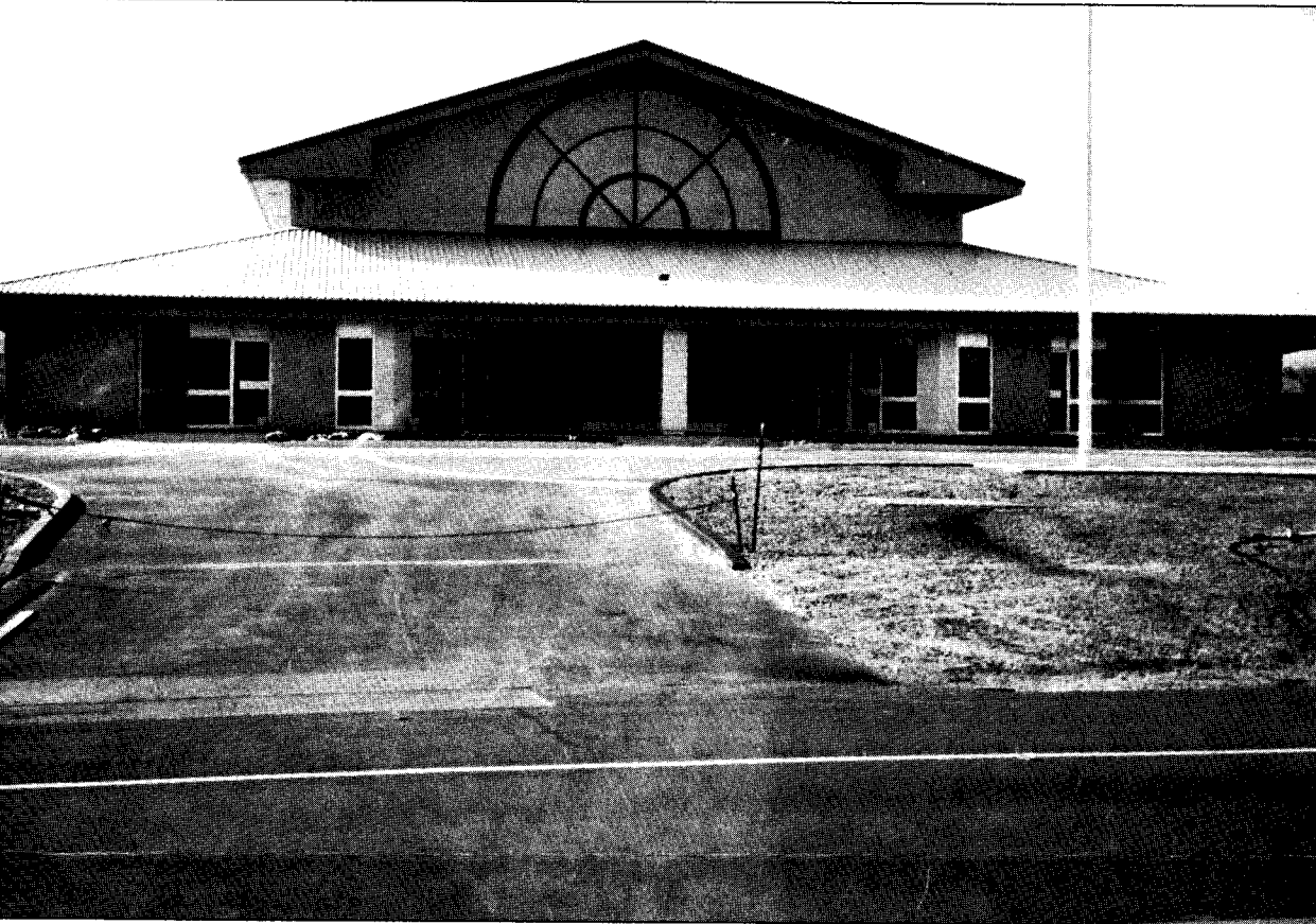
newly-completed Kauai Veterans Center on Kapule Highway, Lihue.
