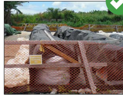
Contaminated material stockpiles must have signage designating material as contaminated.
