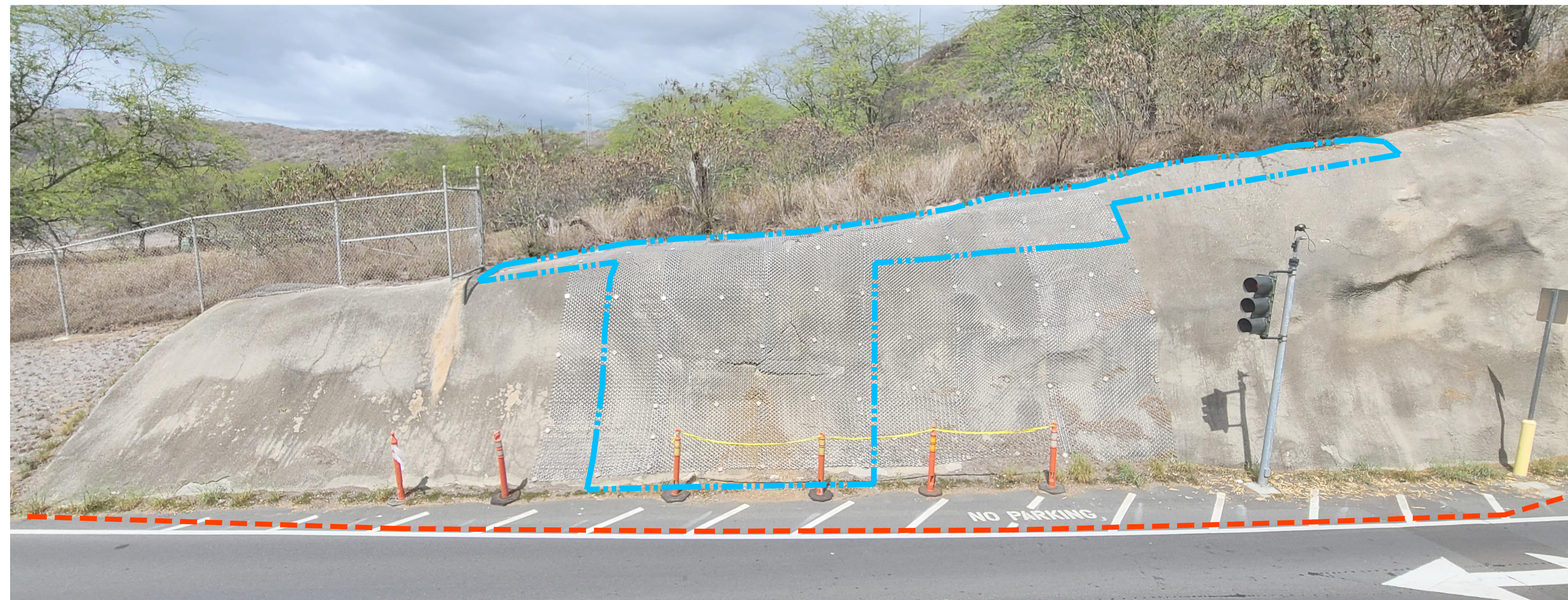
SHOTCRETE WALL REPAIR (DIAMOND HEAD CRATER ROAD)
