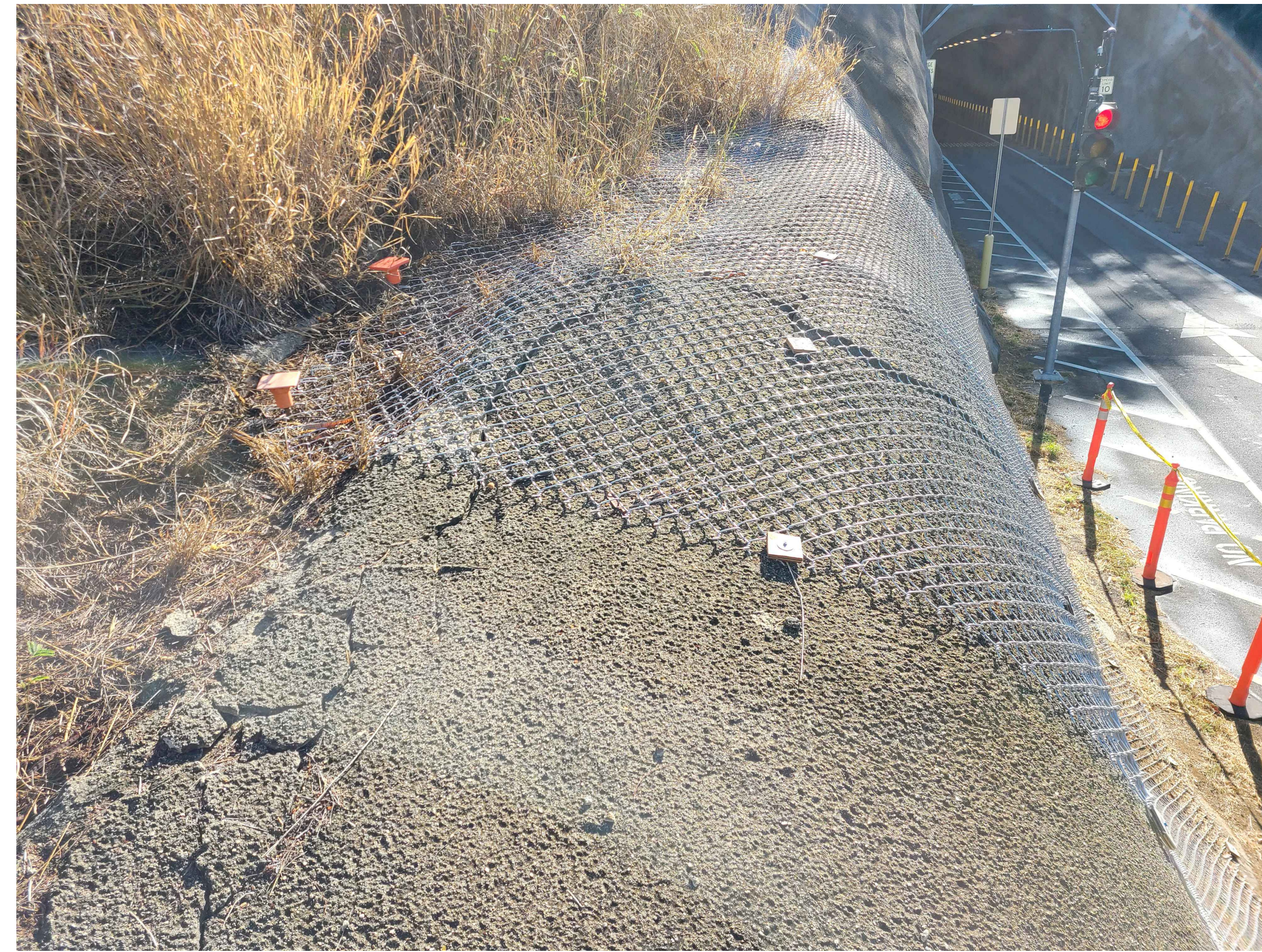
TOP OF NORTH SHOTCRETE WALL
