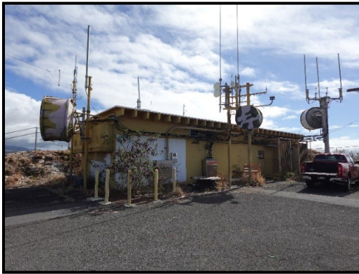
Building PSB October 2023
