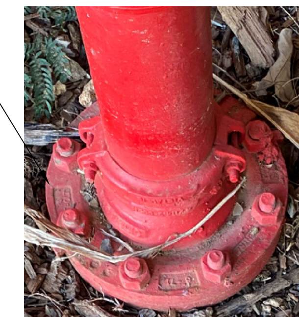
6 B711 CLASSROOM - EXST RISER CONDITION AT GRADE SCALE: NONE
