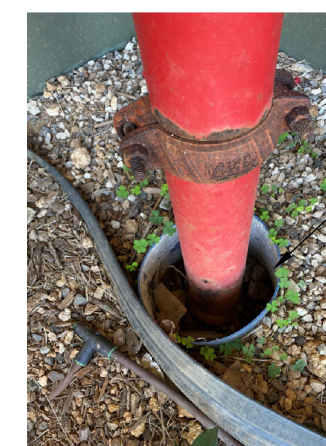
5 B711 ADMIN BLDG - EXST RISER CONDITION AT GRADE SCALE: NONE
