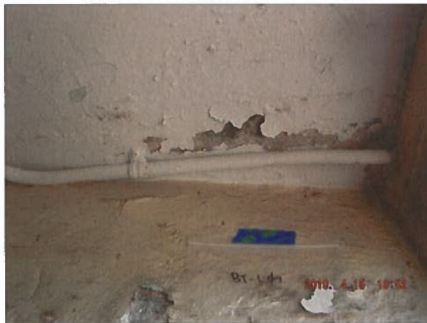
Photo 17 – LCP L-09 (close-up)
