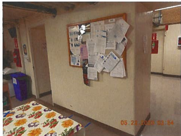
Photo 42 – Non-Lead Dust Hazard W-16
