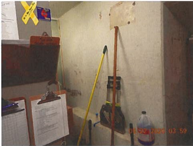
Photo 39 – Lead Dust Hazard W-12
