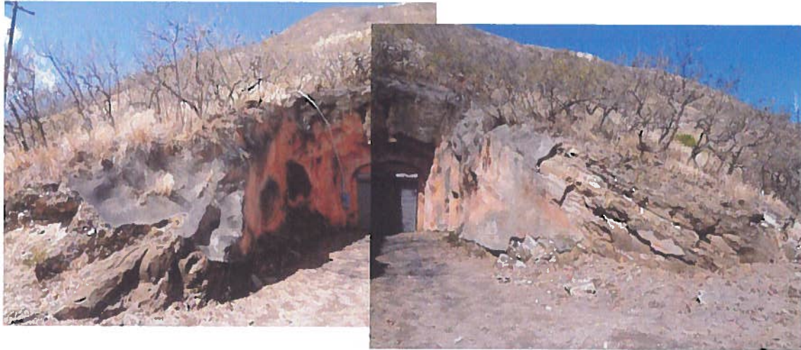
Photographs 4 and 5 – Mule Tunnel 1 non-ACM shotcrete (HSA A2).
