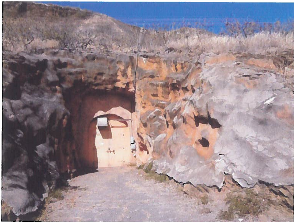
Photograph 9 – Mule Tunnel 3 non-ACM shotcrete (HSA A4).
