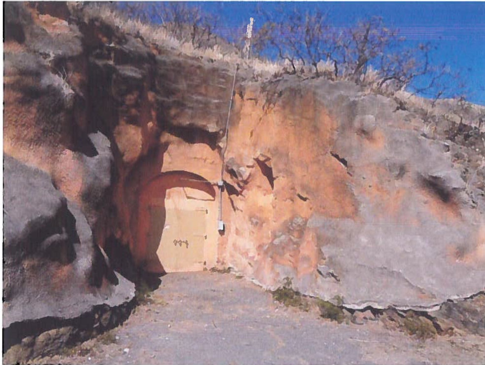
Photograph 7 – Mule Tunnel 2 non-ACM shotcrete (HSA A3).
