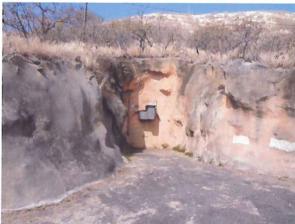
Photograph 11 – Mule Tunnel 5 non-ACM shotcrete (HSA A5).
