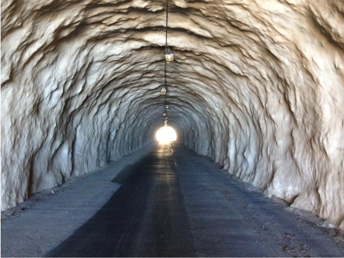
Kapahulu Tunnel, view in the tunnel
