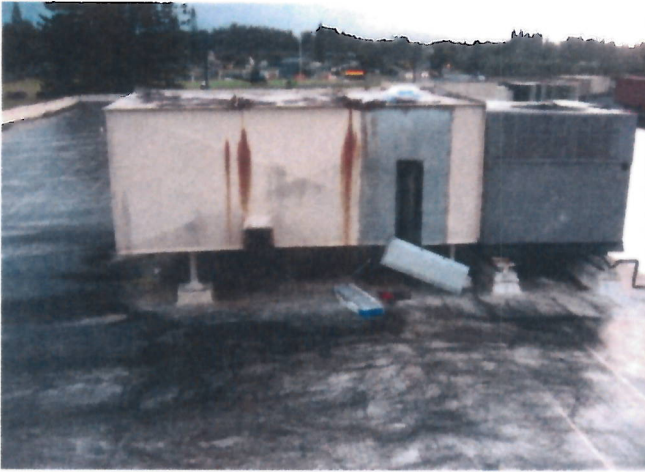
Photograph 1 View of roof-mounted ventilation and air-conditioning unit
