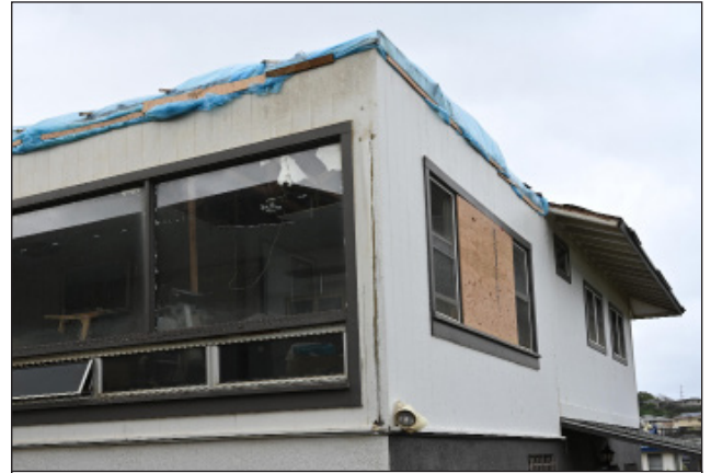
This home on O'ahu lost its roof in the February 2026 Super Bowl weekend storm with sustained winds of 30 to 40 miles per hour. Installing hurricane ties (seen below) likely would have prevented this damage. Photos courtesy Dennis Hwang
