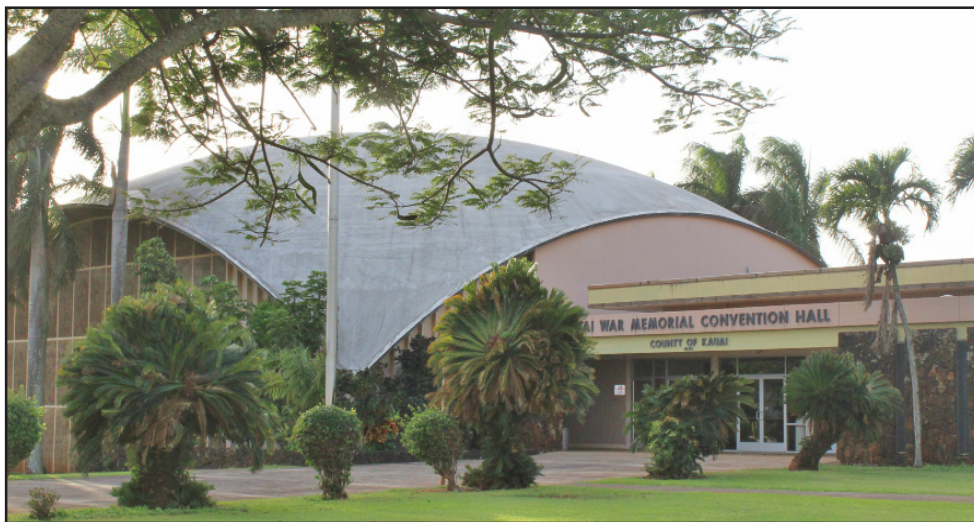
A planned high-wind retrofit of Kaua'i War Memorial Convention Hall in Līhu'e will enable its use as a best available refuge area. Photo courtesy County of Kaua'i
