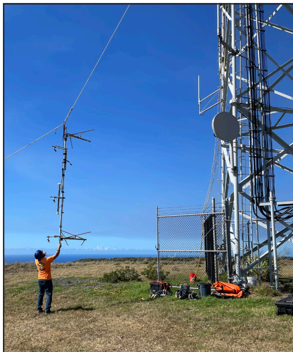
A Coconut Wireless Construction worker lifts the new FM booster antenna onto the Hawai'i County radio tower at South Point.
