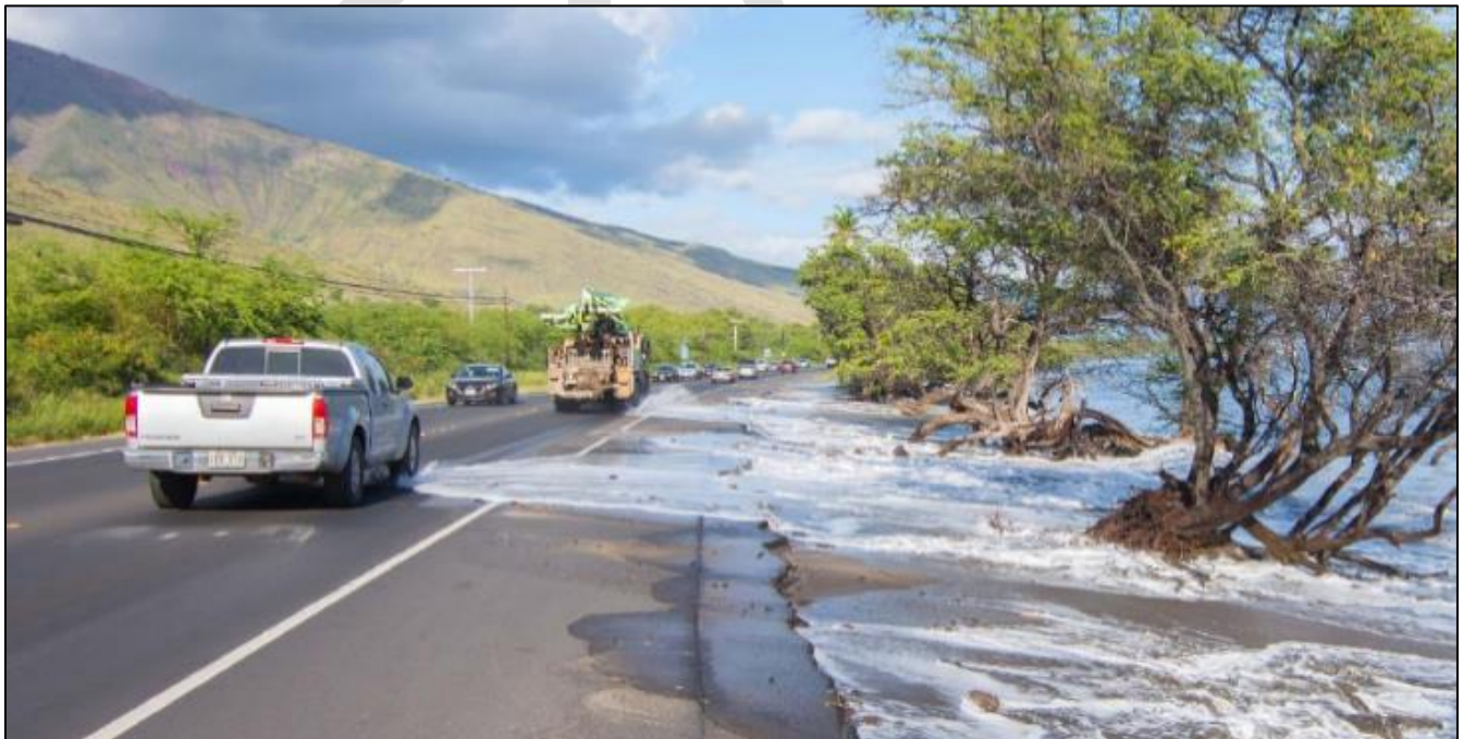
Figure 4.6-4. Wave Inundation at Honoapi'ilani Highway, Maui
