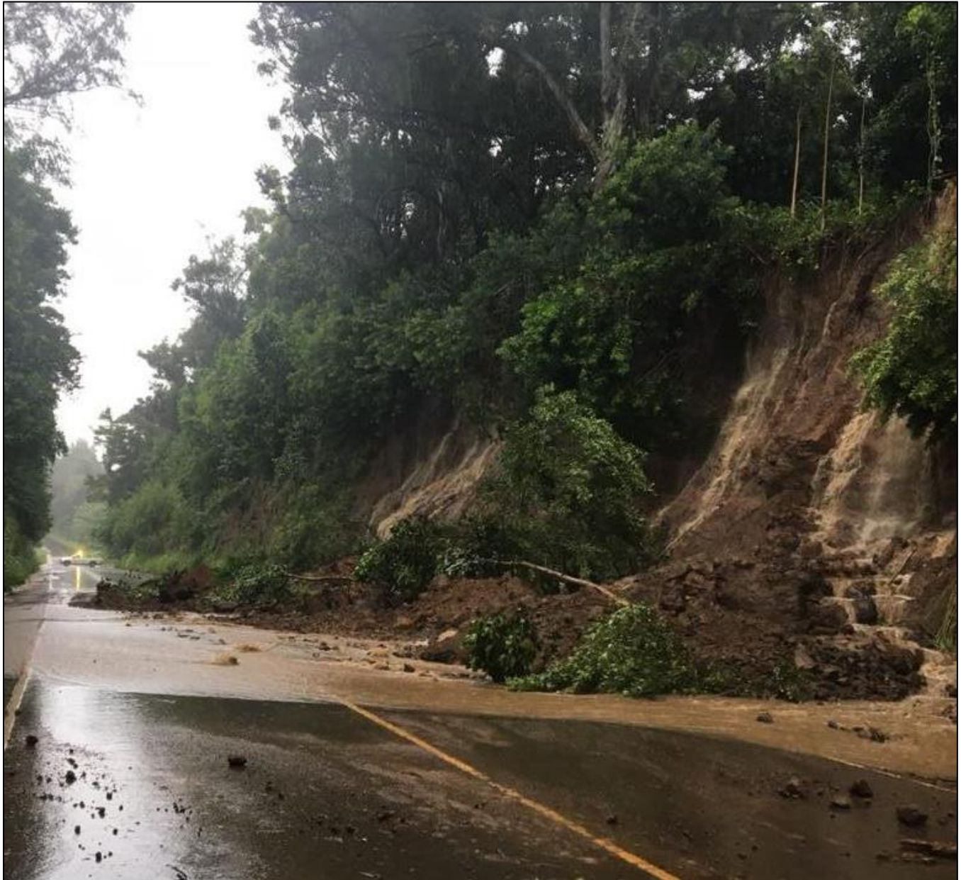
Figure 4.11-4. Landslide on Hawai'i Island, 2018
