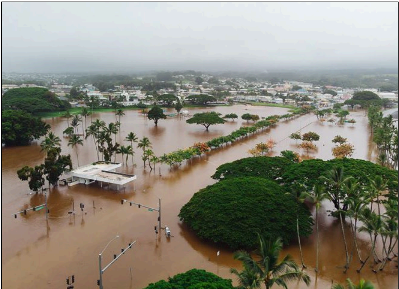
Figure 4.9-2. Flooding in Hilo from Hurricane Lane, 2018
