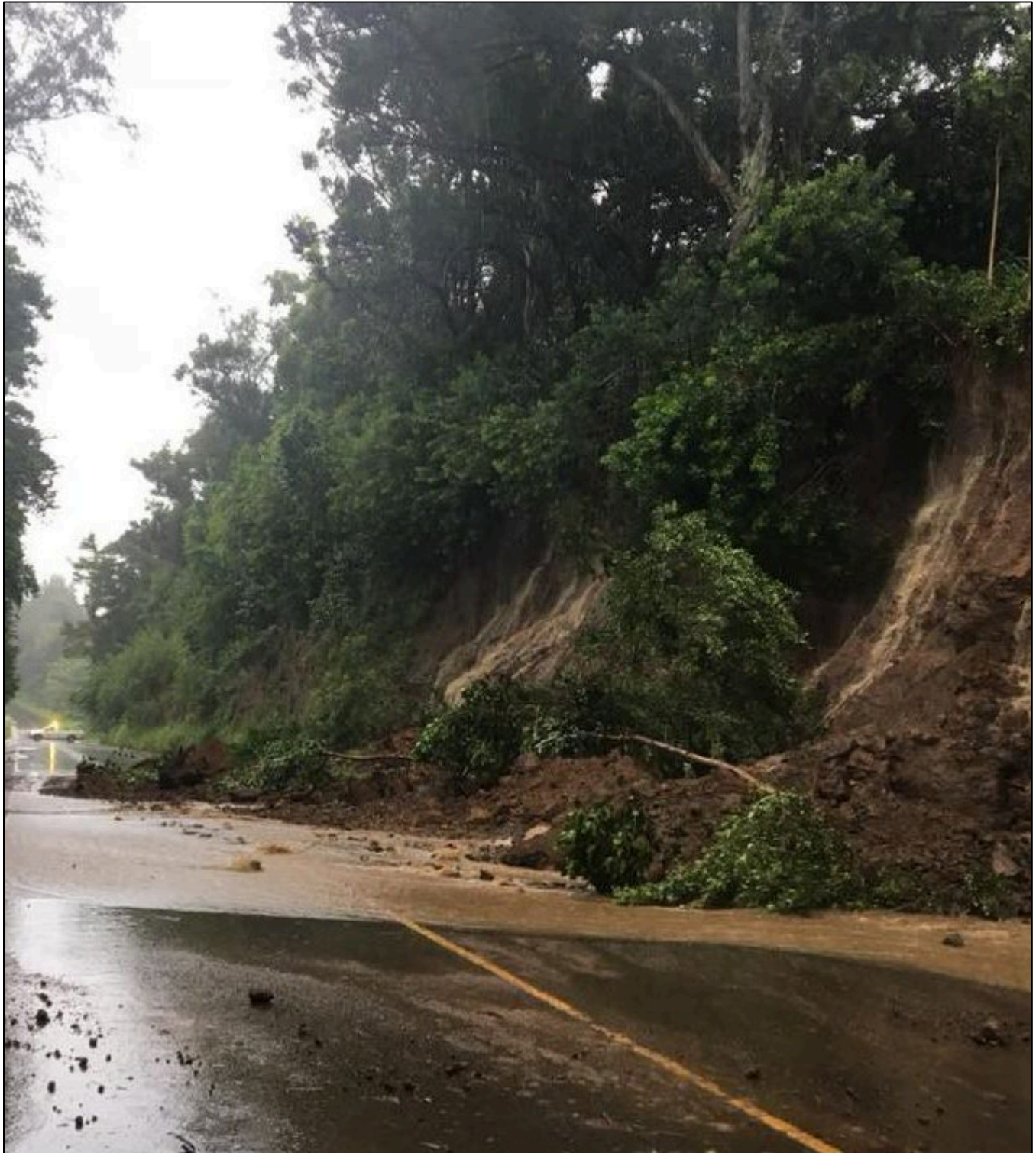
Figure 4.11-8. Landslide on Hawai'i Island, 2018
