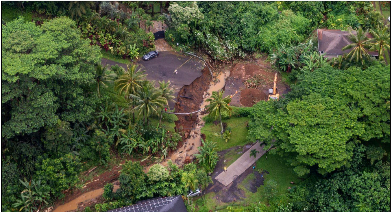
Figure 4.9-3. Road Washout in Maui from Hurricane Lane Flooding
