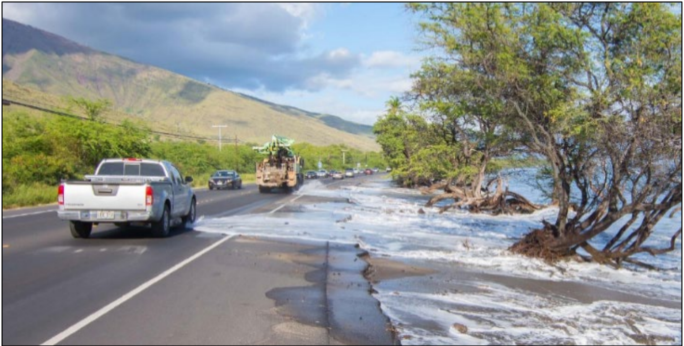
Figure 4.6-4. Wave Inundation at Honoapi'ilani Highway, Maui
