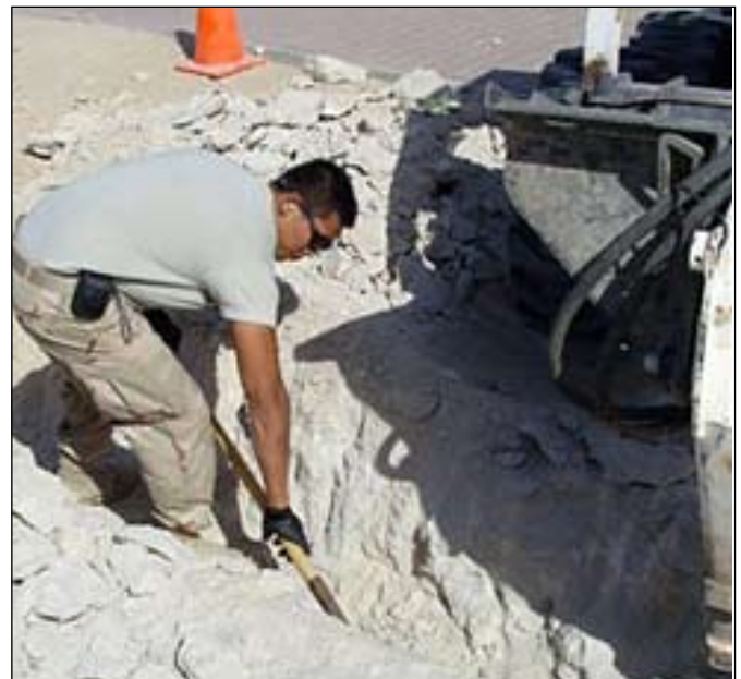
(T-L) Master Sgt. Darren Atabay digs a trench to install communications lines in a remote area in Kuwait.
