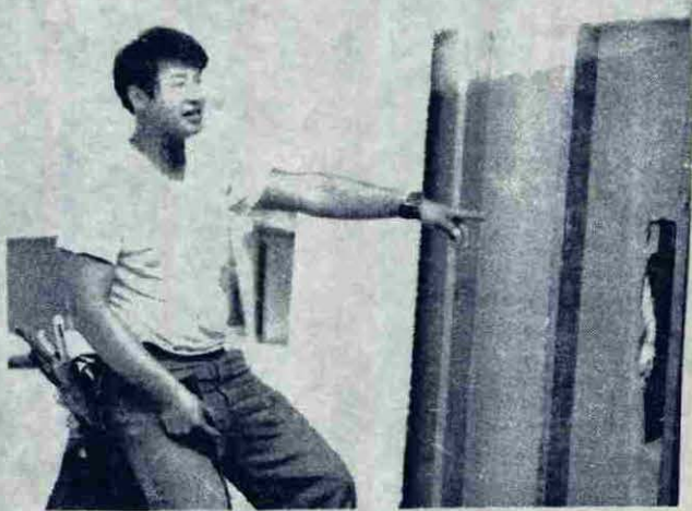
HARD WORKING ELECTRICIAN: SSgt Calvin Ko points to electrical conduit in the old HANG hangar where the 154th Civil Engineering Flight is hard at work. HANG Photo by Sgt. Donald Ho.
