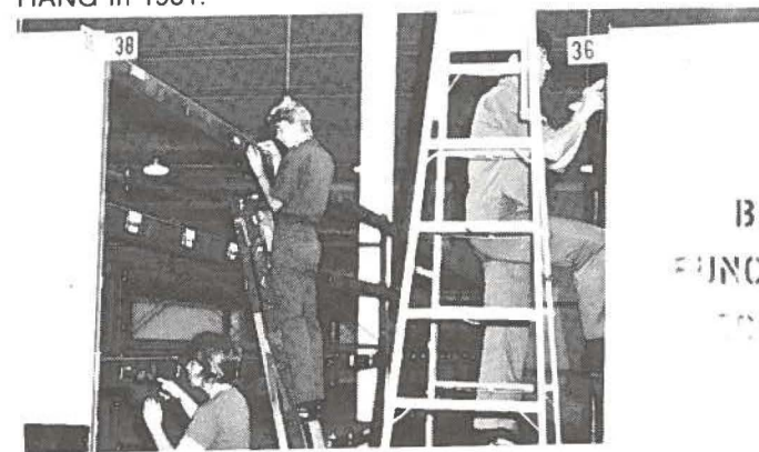
RMS members are constantly busy maintaining and documenting HANG resources. Workers here prepare a new storage area.
