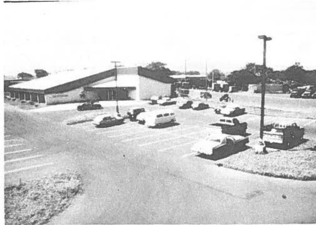
201st CCFT electronic maintenance facility at Kahului, Maui.
