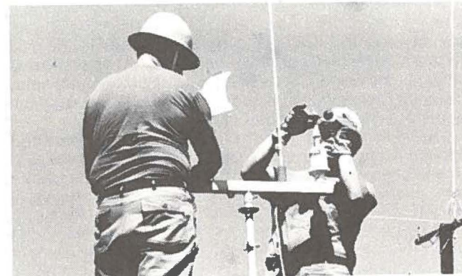
ATC personnel install wind speed/direction indicators for AN/TSW-7.
