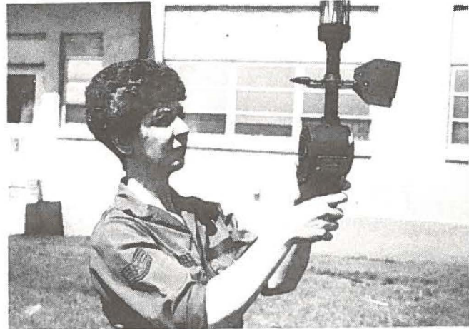
SSgt. Jean Burrell checks wind velocity & direction with the anemometer.
