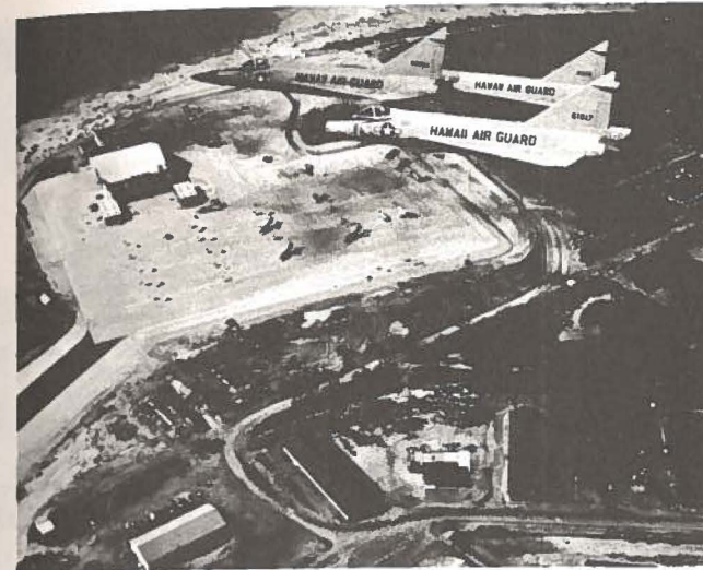
NEW HOME. The new fighter facility at Fort Kamehameha.
