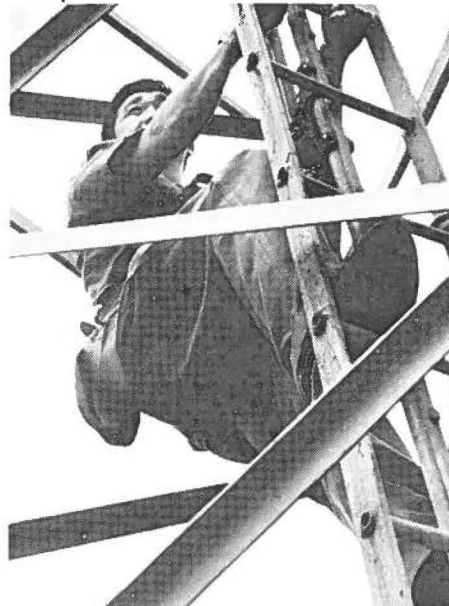
TSgt Gerald J. Yamamoto climbing the 180' Microwave Tower atop Mt. Kaala.
